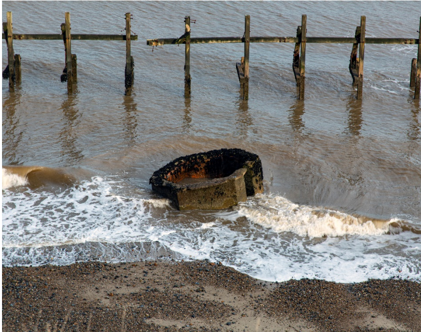
Alan D Horn Happisburgh North Norfolk Nov 2019 Pill Box fallen into the sea – a result of recent cliff fall
